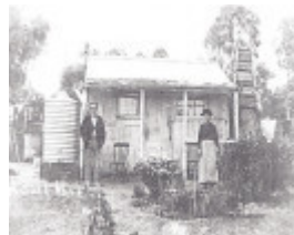
Miners Timber Slab Cottage 2 Castle Rd Black & White 1 - Shire of Eltham Heritage Study 1992
