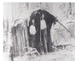
Miners Timber Slab Cottage 2 Castle Rd Black & White 2 - Shire of Eltham Heritage Study 1992
