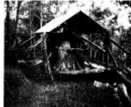
31 - Miners Timber Slab Cottage 2 Castle Rd - Shire of Eltham Heritage Study 1992
