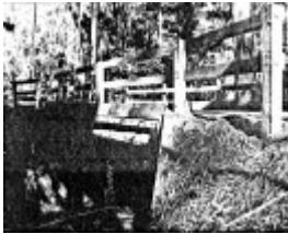
33 - Timber Trestle Road Bridge over Arthurs Creek - Shire of Eltham Heritage Study 1992
