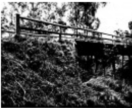
34 - Timber Trestle Road Bridge Chapel Lane_02 - Shire of Eltham Heritage Study 1992
