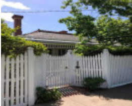
3 Seymour Avenue, Armadale
