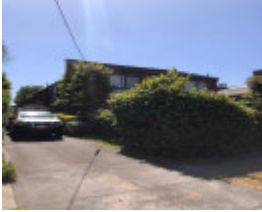
27 Seymour Avenue, Armadale
