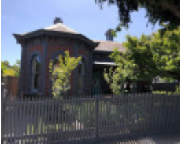
31 Seymour Avenue, Armadale
