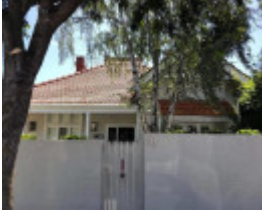
35 Seymour Avenue, Armadale
