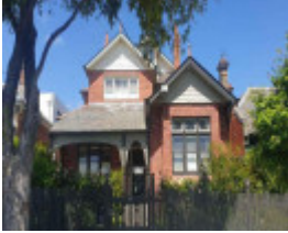
16 Seymour Avenue, Armadale
