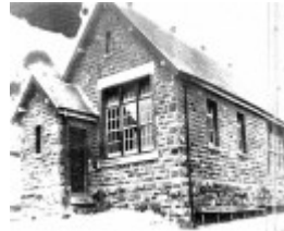
50 - Eltham Primary School Dalton St - Early 20th century photograph taken after the installation of larger windows, a process undertaken at many Victorian State Schools at that time. Note the smaller windows, which are presumably original (ELHPC No.642)
