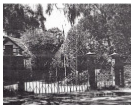
Adobe Residence and Iron Gates 25 Diamond St_03 - Shire of Eltham Heritage Study 1992
