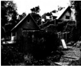
53 - Adobe residence and Batemans Studio 57 Dodd St - Shire of Eltham Heritage Study 1992
