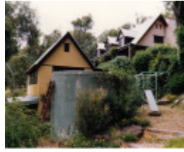
Adobe residence and Batemans Studio 57 Dodd St Colour 6 - Shire of Eltham Heritage Study 1992
