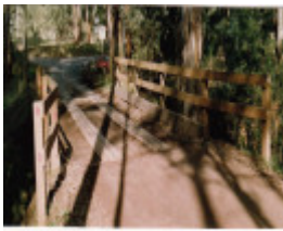
Timber Trestle Bridge Arthurs Creek Eagles Nest Rd Colour 4 - Shire of Eltham Heritage Study 1992
