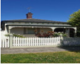
32 Seymour Avenue, Armadale
