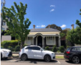
42 Lambeth Avenue, Armadale
