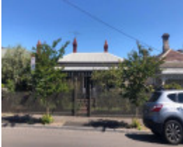
17 Llaneast Street, Armadale
