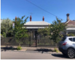
17 Llaneast Street, Armadale
