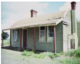
gordon railway station gowrie street gordon front view nov1986
