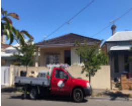
23 Llaneast Street, Armadale
