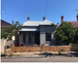
25 Llaneast Street, Armadale
