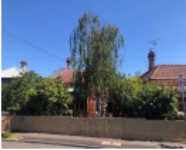
27 Llaneast Street, Armadale
