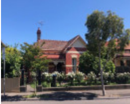
29 Llaneast Street, Armadale
