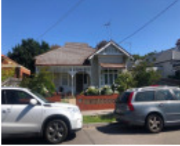
37 Llaneast Street, Armadale
