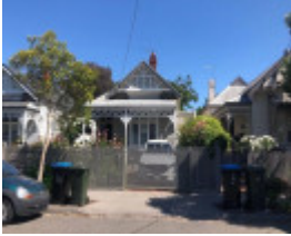
41 Llaneast Street, Armadale
