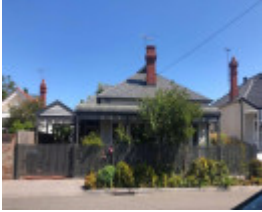
47 Llaneast Street, Armadale
