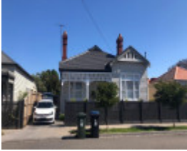
49 Llaneast Street, Armadale
