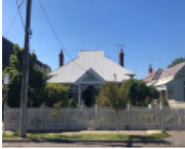
56 Llaneast Street, Armadale
