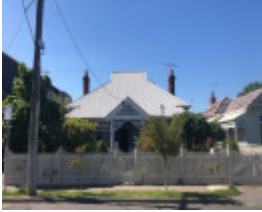
56 Llaneast Street, Armadale
