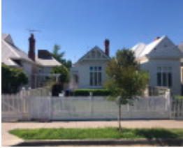
54 Llaneast Street, Armadale
