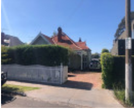
48 Llaneast Street, Armadale
