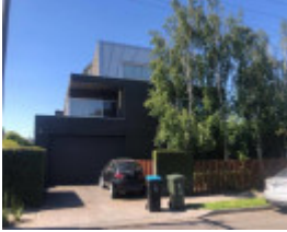
44-46 Llaneast Street, Armadale
