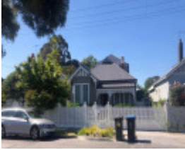
40 Llaneast Street, Armadale
