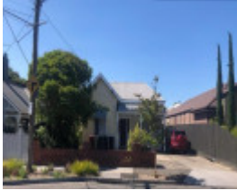
36 Llaneast Street, Armadale
