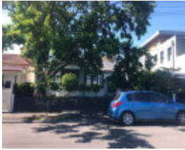
14 Llaneast Street, Armadale
