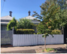
22 Llaneast Street, Armadale
