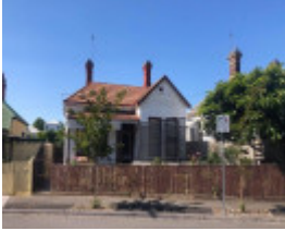
30 Llaneast Street, Armadale
