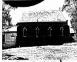
63 - Presbyterian Church Eltham Yarra Glen Rd_03 - Shire of Eltham Heritage Study 1992
