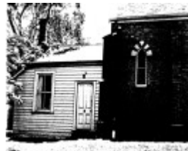
63 - Presbyterian Church Eltham Yarra Glen Rd_05 - Shire of Eltham Heritage Study 1992
