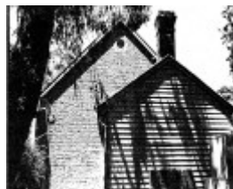
63 - Presbyterian Church Eltham Yarra Glen Rd_09 - Shire of Eltham Heritage Study 1992
