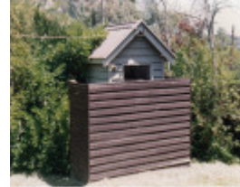
Kangaroo Primary State School Elth Yarr Glen Rd Colour 6 - Shire of Eltham Heritage Study 1992
