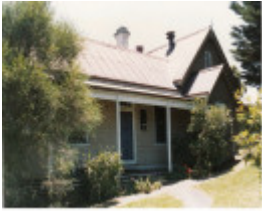
Kangaroo Primary State School Elth Yarr Glen Rd Colour 2 - Shire of Eltham Heritage Study 1992
