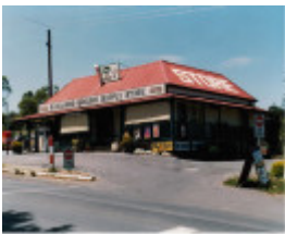
Kangaroo Ground General Store Post Office Pines Colour 6 - Shire of Eltham Heritage Study 1992
