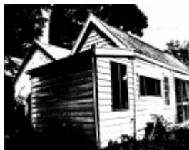
69 - Garden Hill Shearing Shed Elth Yarra Glen Rd - Shire of Eltham Heritage Study 1992
