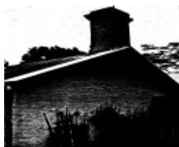
69 - Garden Hill Shearing Shed Elth Yarra Glen Rd_06 - Shire of Eltham Heritage Study 1992
