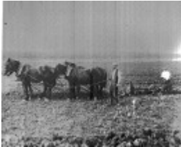
69 - Garden Hill Shearing Shed Elth Yarra Glen Rd_13 - James and Robert Ness ploughing at Garden Hill (ELHPC NO. 420) - Shire of Eltham Heritage Study 1992
