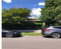
50 Stuart Street, Armadale
