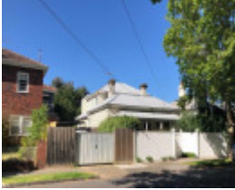
6 Union Street, Armadale
