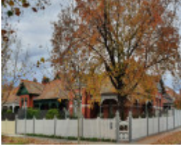
10 Union Street, Armadale
