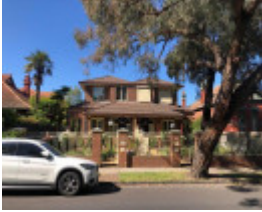
18-18A Union Street, Armadale
