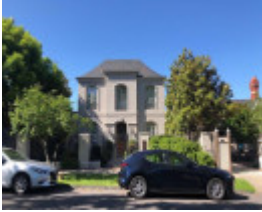
36 Union Street, Armadale
