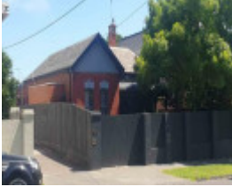
38 Union Street, Armadale
