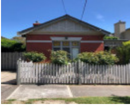
50 Union Street, Armadale
