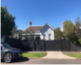
62 Union Street, Armadale
