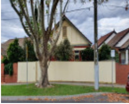
1 Union Street, Armadale
