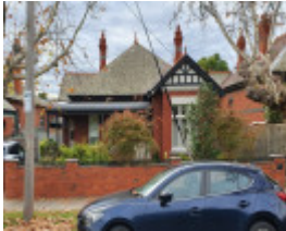
23 Union Street, Armadale
