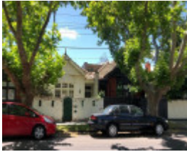
31-33 Union Street, Armadale
