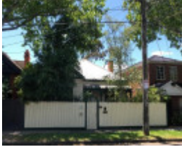
35 Union Street, Armadale
