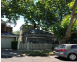
39 Union Street, Armadale
